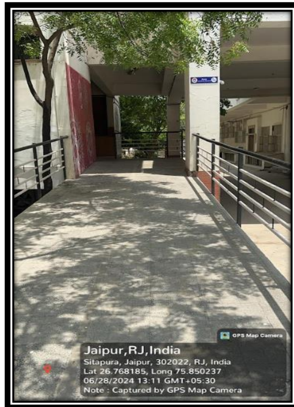
Picture 1: Ramp with Rails for academic Block- A
